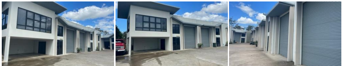
3-5 Enterprise Cct, Maryborough West
