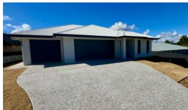
37 Excalibur Crescent, Southside
