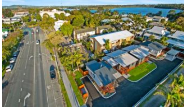
4, 79 Poinciana Avenue, Tewantin
