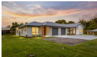
25a Mill St, Landsborough
