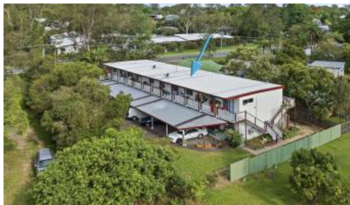
Unit 9, 28 Kauri St, Cooroy
