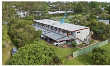
Unit 9, 28 Kauri St, Cooroy
