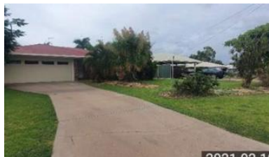
2 Cowan Crescent, Emerald
