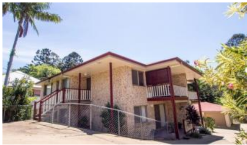
1, 26 Blackall Terrace, Nambour
