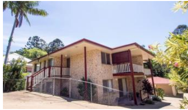
1, 26 Blackall Terrace, Nambour
