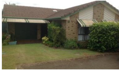
10, 15 Townsend Road, Buderim
