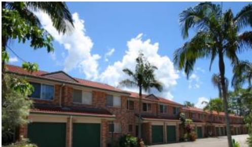
4, 76 Blackall Terrace, Nambour
