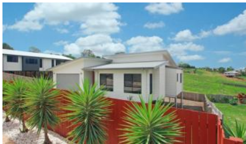
27 Moss Day Place, Burnside
