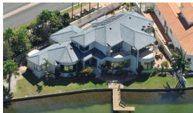
21 Saltwater Avenue, Noosaville
