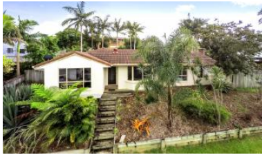
25 Orlando Crescent, Kuluin
