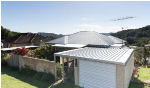
45 Lamington Terrace, Nambour
