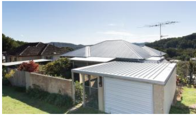
45 Lamington Terrace, Nambour
