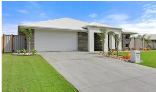
19 Seahaven Cct, Pialba
