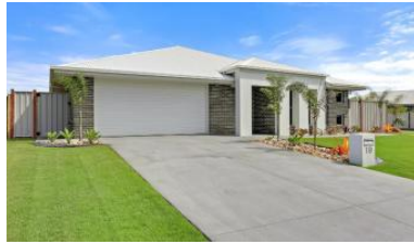
19 Seahaven Cct, Pialba
