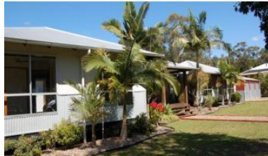
23 Coolah Place, Cooroibah
