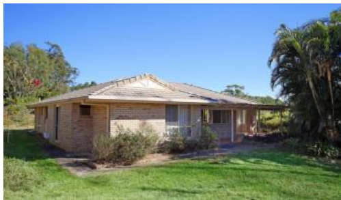
13 Curlew Crescent, Cooroy
