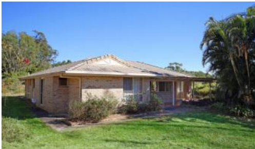
13 Curlew Crescent, Cooroy
