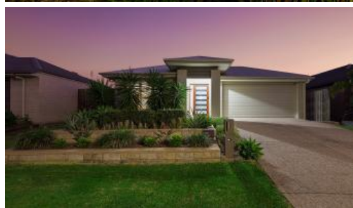
17 Keppel St, Meridan Plains
