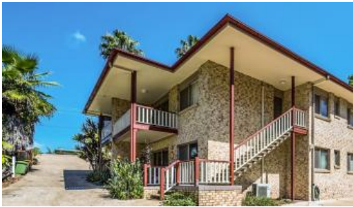
Unit 1, 26 Blackall Tce, Nambour
