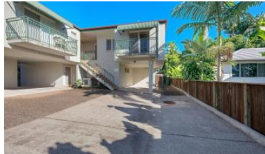
Unit 8, 5 Vernon St, Nambour
