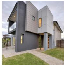
7 Reserve Court, Murrumba Downs
