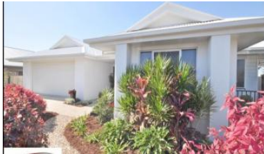
18 Rawlins Crescent, North Lakes
