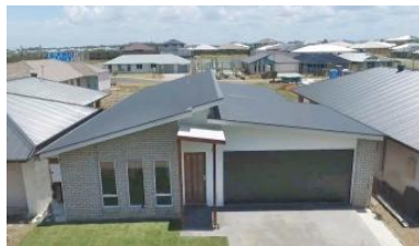
20 Southwood Court, Mango Hill
