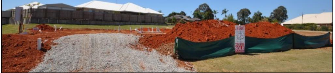
Lot 40, 4 Hugh Crescent, Murrumba Downs
