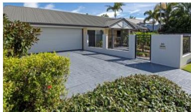
80 Lamerough Pde, Pelican Waters
