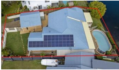
76 Lamerough Pde, Pelican Waters
