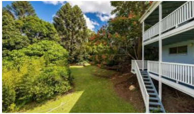
1, 59 Blackall Terrace, Nambour
