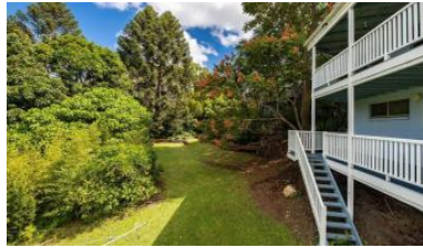
1, 59 Blackall Terrace, Nambour
